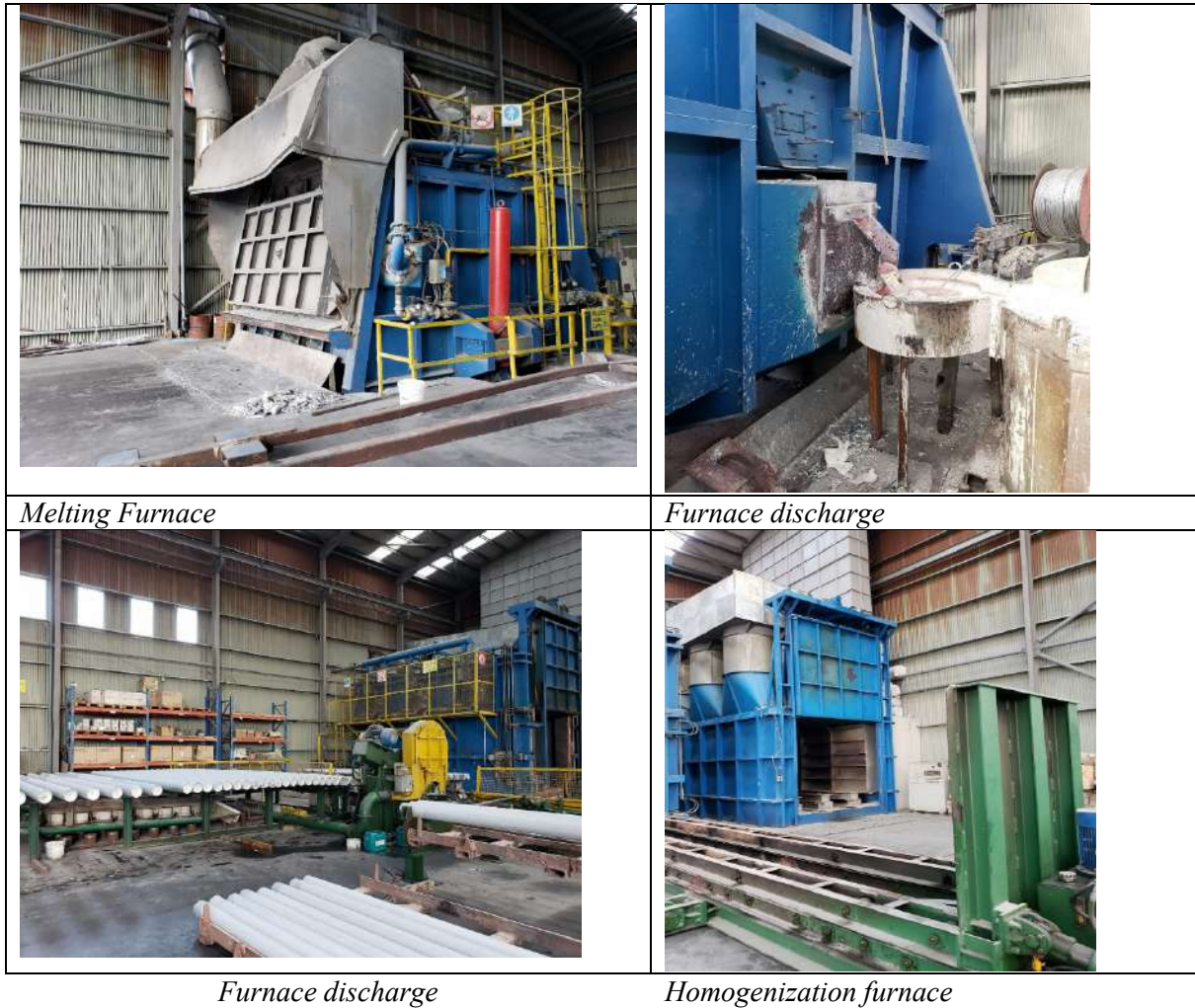
Figure 5: Aluminium Recycling equipments technology in Everest industry in Albania
